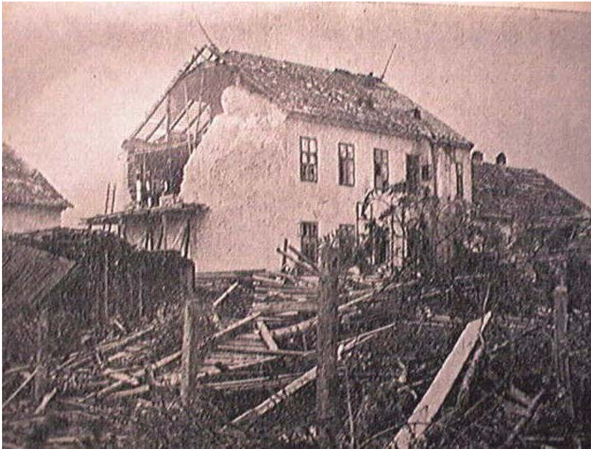
Badly damaged house, Wr. Neustadt 1916 (Bild von www.tornados.at )
